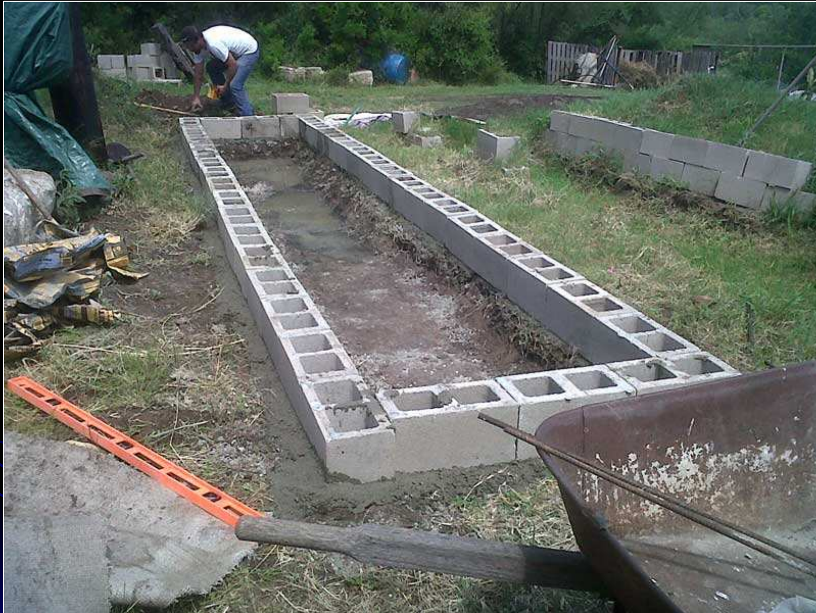
First row of retaining wall completed using 8" x 16" cinder blocks
