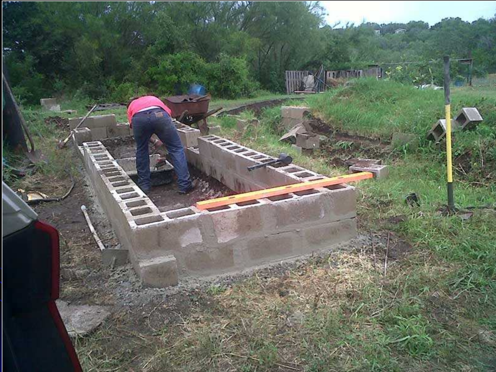
Building second row of retaining wall
